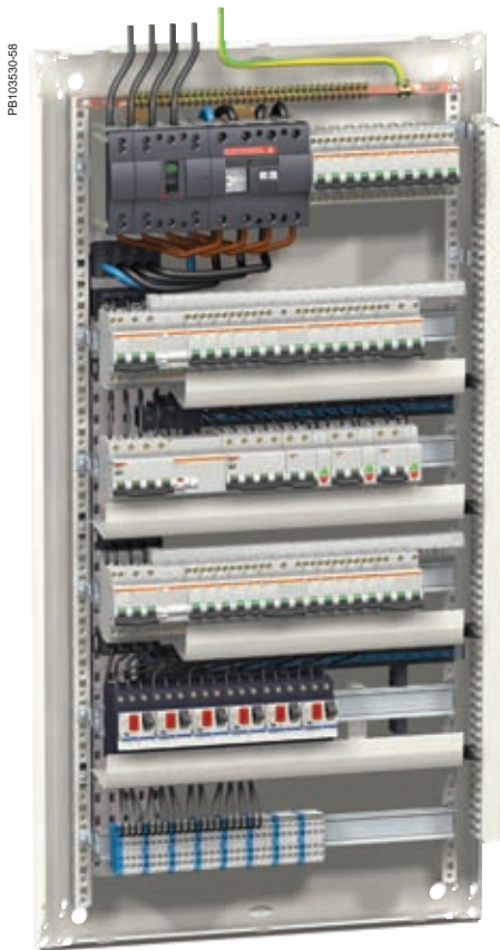
NG160 in modular enclosure.
